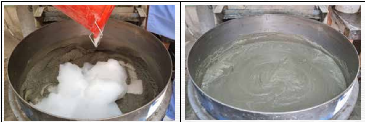
Figure 5-10 Adding foam to mortar (left) and mixed foamed concrete (left)
