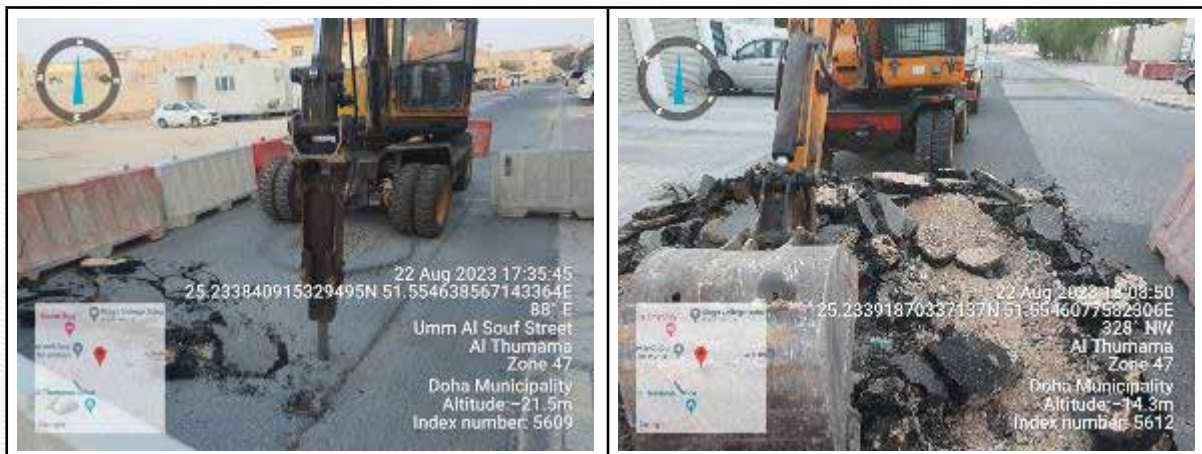
Figure 7-7 Excavation around manhole cover
