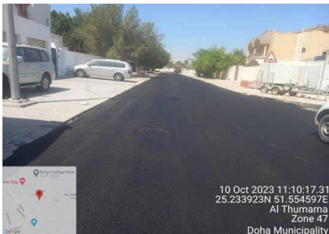
Figure 7-12 Placing the new asphalt wearing course on top of foam concrete
