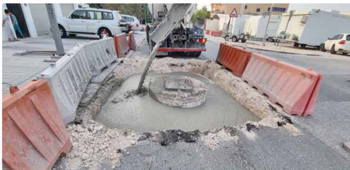
Figure 7-9 Application of PC foamed concrete around manhole cover
