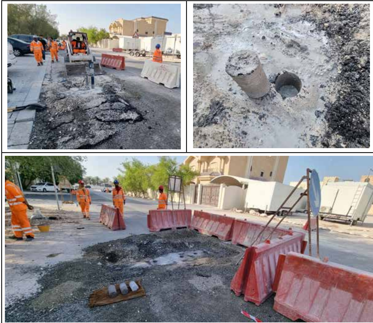
Figure 7-15 Coring of foam concrete around manhole covers
