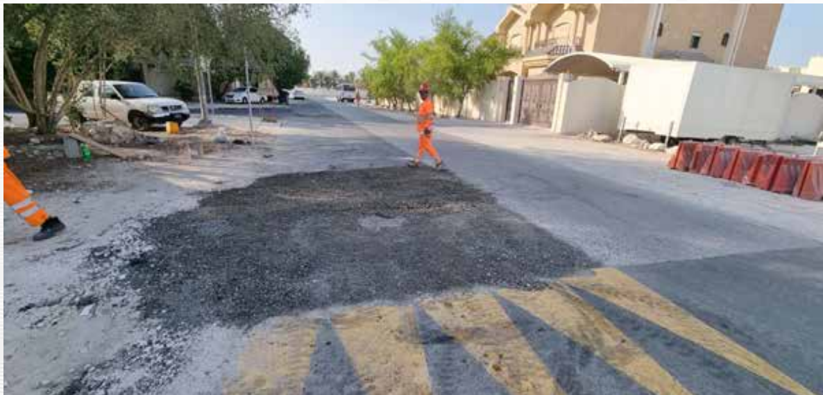
Figure 7-11 Covering of foam concrete with RAP
