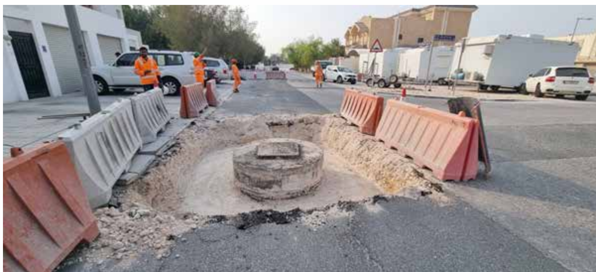
Figure 7-8 Completed excavation around manhole cover
