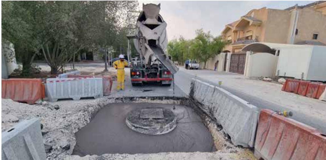
Figure 7-10 Application of SSA foamed concrete around manhole cover
